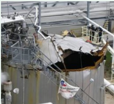
Ruptured sulphur tank
