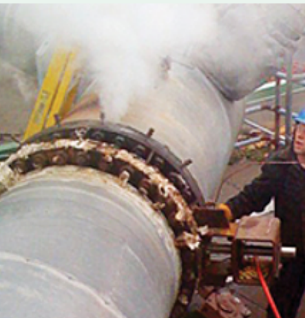
Re-injection on a clamp on leaking flange.
